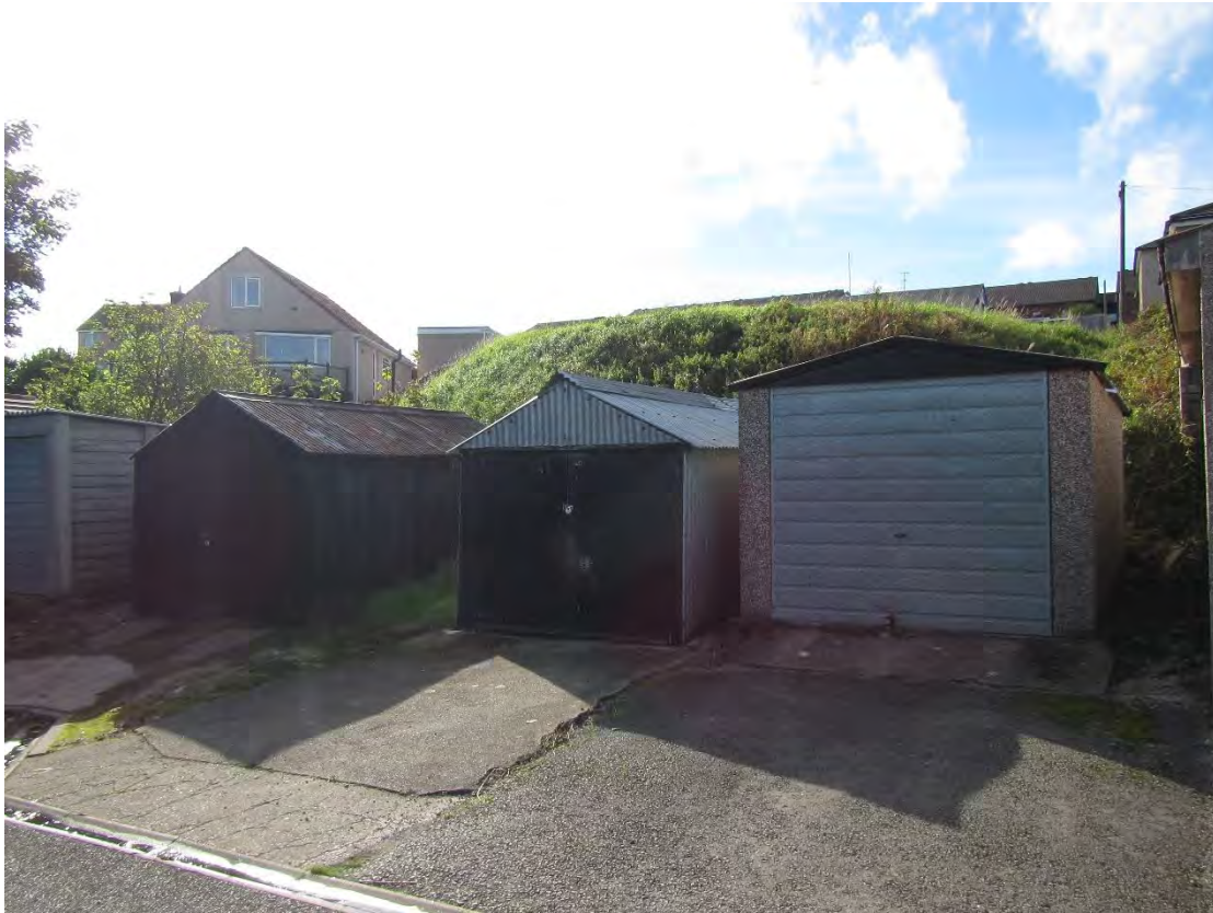
Photograph 6 – Looking west towards buildings 5, 6 and 7.
