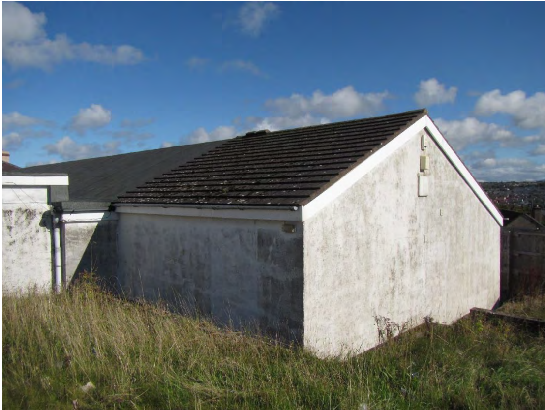
Photograph 2 – Looking north-east towards building 1.
