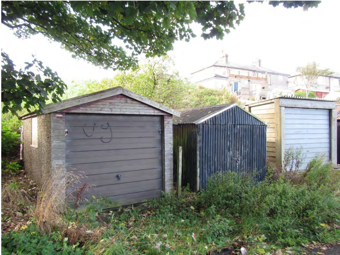
Photograph 5 – Looking west towards buildings 2, 3 and 4.
