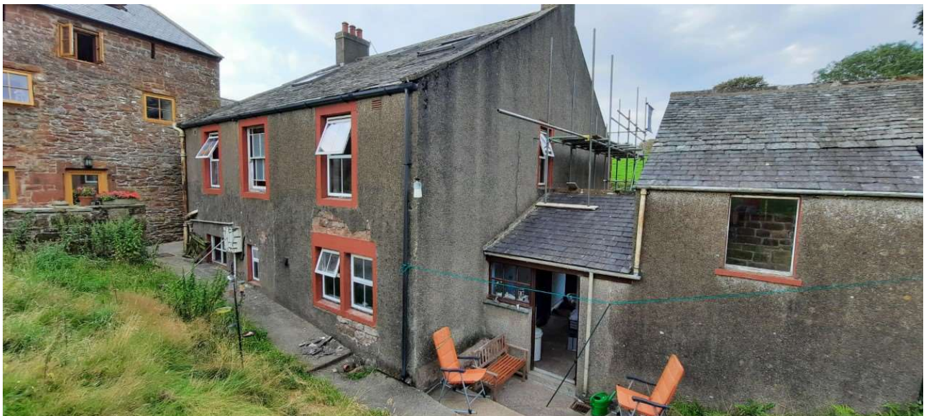
Photo showing rear and south side elevation of main house ('Bothy' visible to right)
